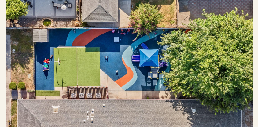
Reconstructed play yard surfacing and turf, completed 2024
